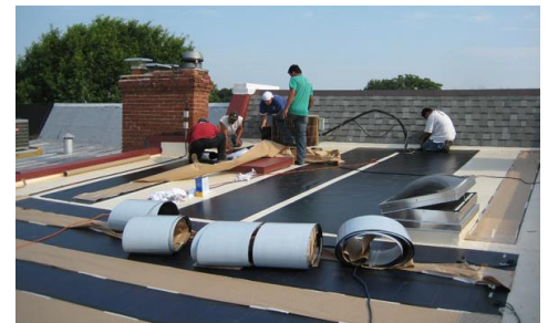
Installation Underway on Mt. Pleasant Rooftop Source: Mt. Pleasant Solar Co-op
